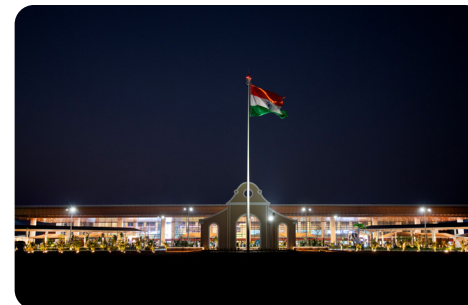
Goa International Airport, India
