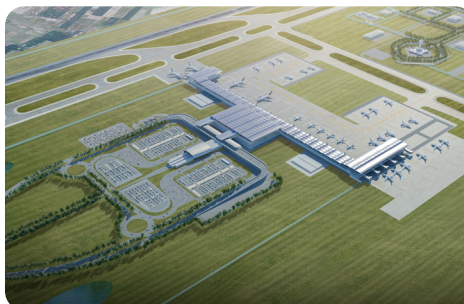
Kualanamu International Airport, Indonesia
