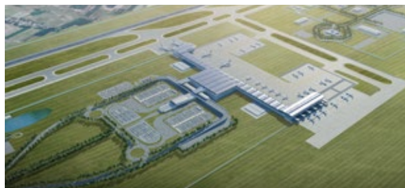
Kualanamu International Airport, Indonesia
