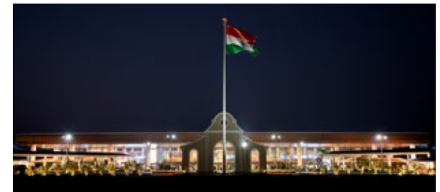
Goa International Airport, India
