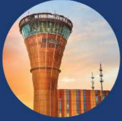
Goa International Airport, Mopa, Goa, India
