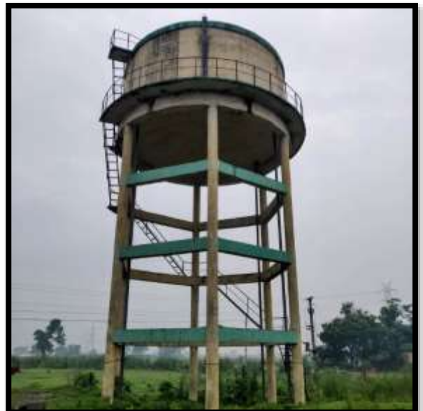
FIGURE 24: WATER STORAGE TANK, MANPUR
