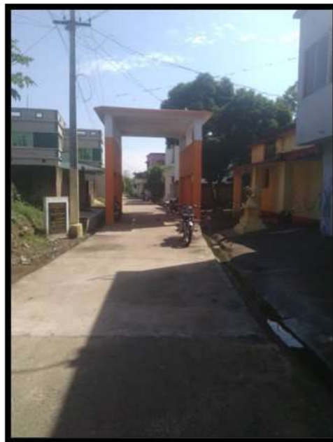
FIGURE 22: CONCRETE ROAD INSIDE MANPUR VILLAGE
