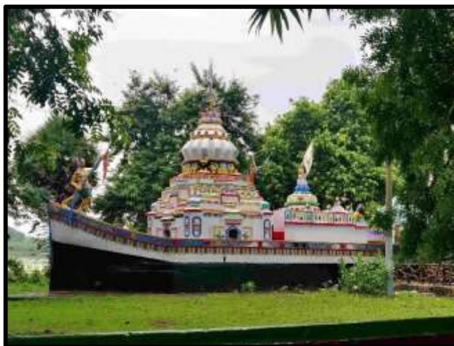
FIGURE 26: TEMPLE RENOVATION, KAMALANGA
