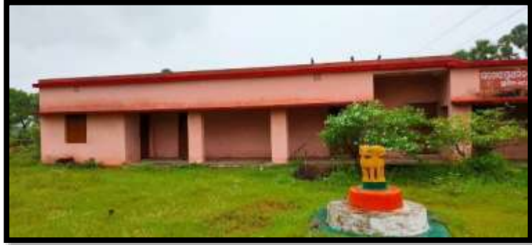
FIGURE 23: RENOVATED SCHOOL BUILDING
